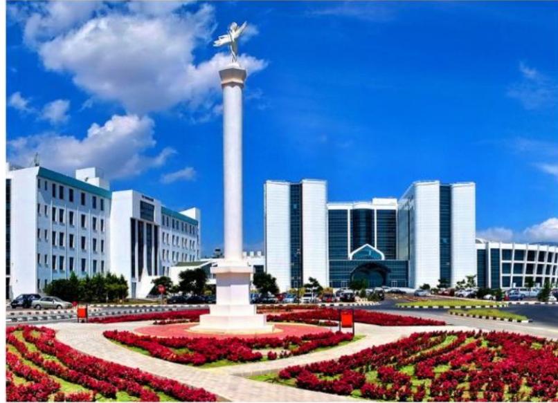
NEAR EAST UNIVERSITY HOSPITAL (LEFKOŞA)
