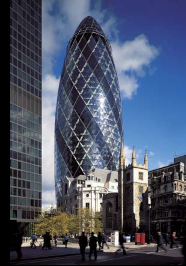
Swiss Re Headquarters, UK
